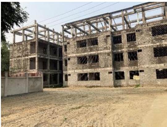
Figure 4: 4 storeyed under-construction building of Palli Janapad
