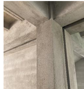
Figure 8: Expansion joint among column
