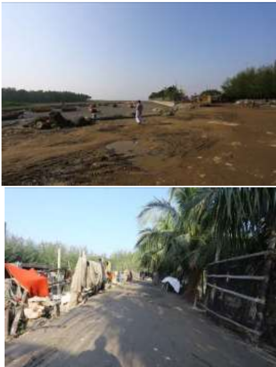
Figure 5- Fragile condition of Embankment
