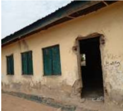
Plate 9: Showing Damaged Door
