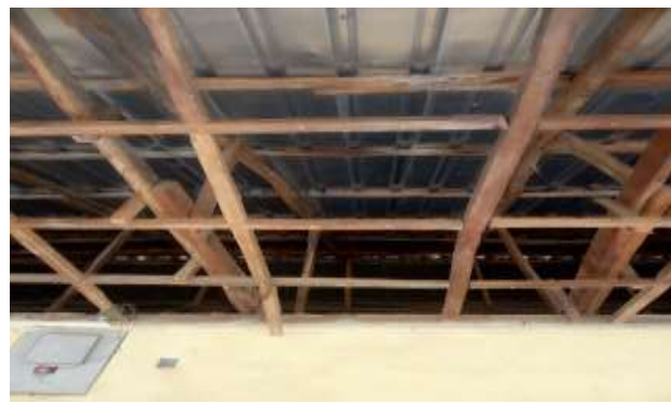
Plate 2: Showing corridor without ceiling
