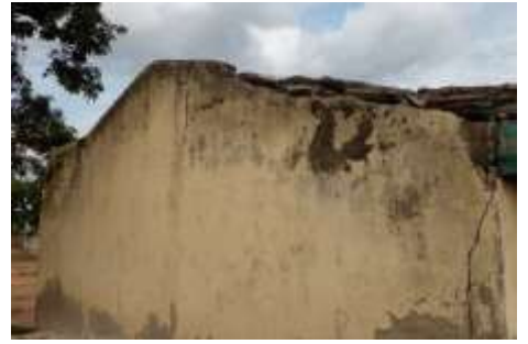
Plate 12: Showing dilapidated eaves and parapet
